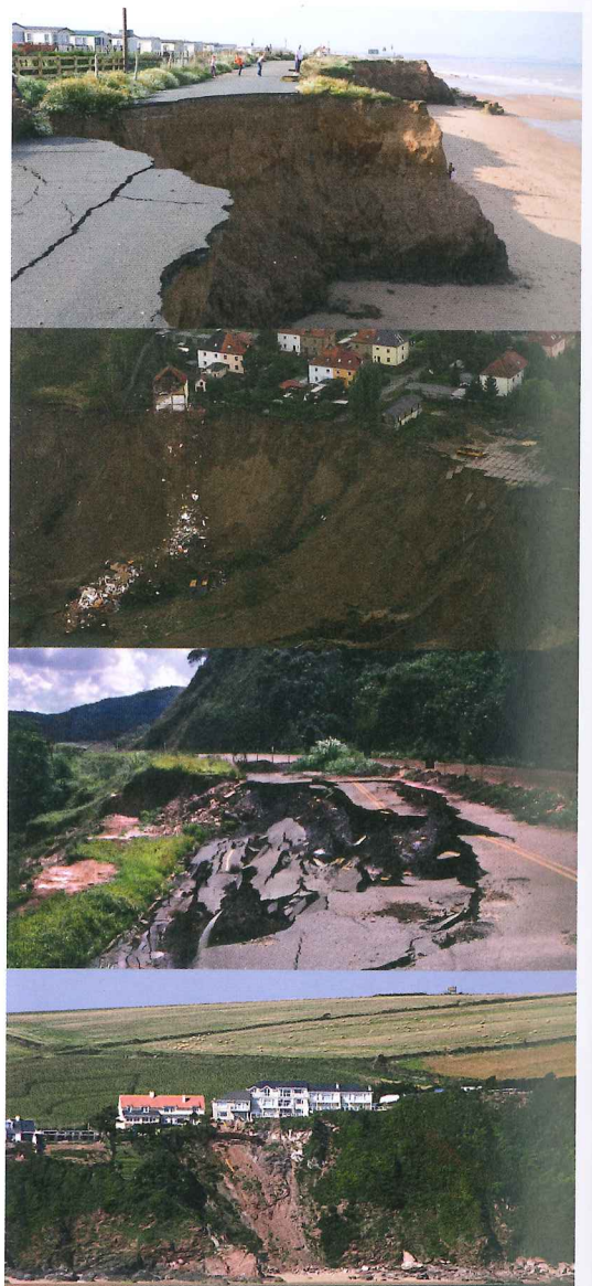
Figure 2.36 Soil erosion can lead to many problems.
