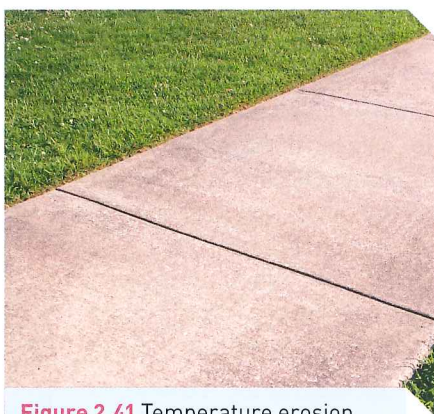
Figure 2.41 Temperature erosion causes materials such as concrete to crack. Footpaths have grooves in them to allow for their expansion during hot weather.
