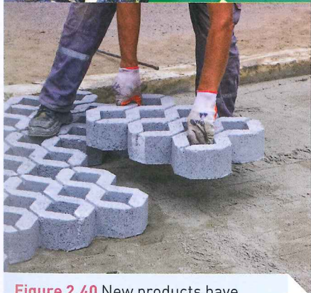
Figure 2.40 New products have been developed that allow water to move through instead of contributing to run-off. This allows the water to be absorbed into the soil and join the groundwater.
