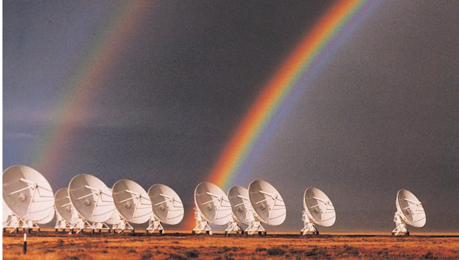
The Very Large Array in New Mexico consists of 27 dishes, each with a diameter of 25 metres, arranged in a 'Y' shape. This is the equivalent of a single radio telescope with a diameter of 35 kilometres.
