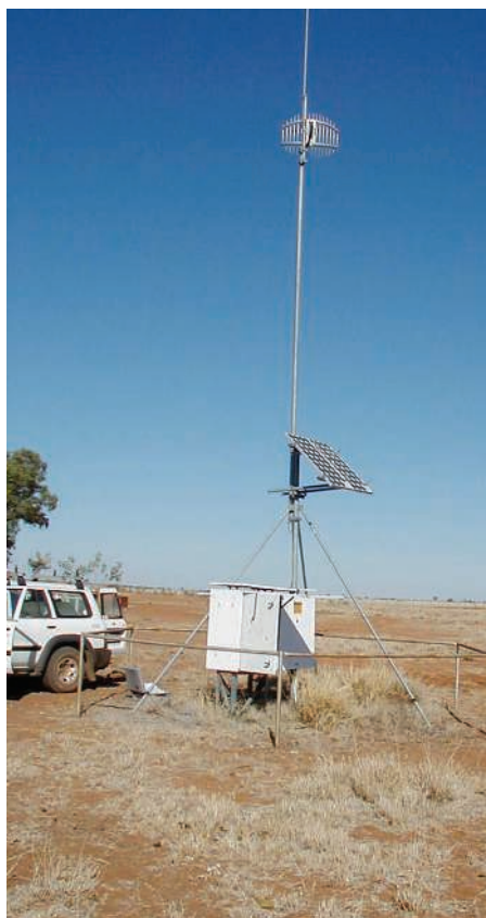
A combined HCRC/DRCS unit being installed
