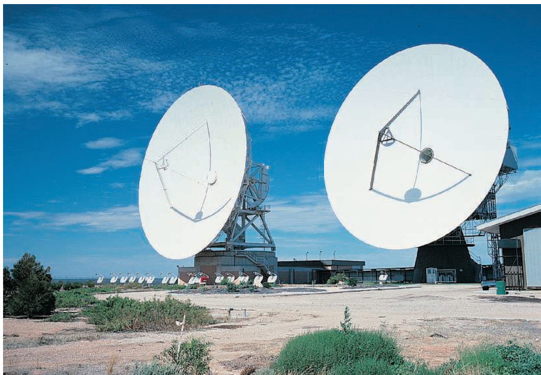
These antennas receive signals that have been retransmitted by a geostationary satellite.
