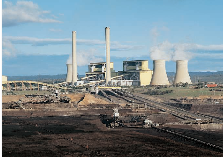
Loy Yang power station in the Latrobe Valley. Victorian coal-fired power stations are built close to open-cut coalmines. Coal is burned to boil water. The resulting high pressure steam is used to drive huge turbines like the ones in the photograph on page 102.
