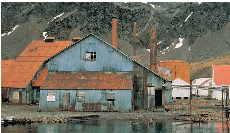
The rusting of this shed is an example of corrosion.
